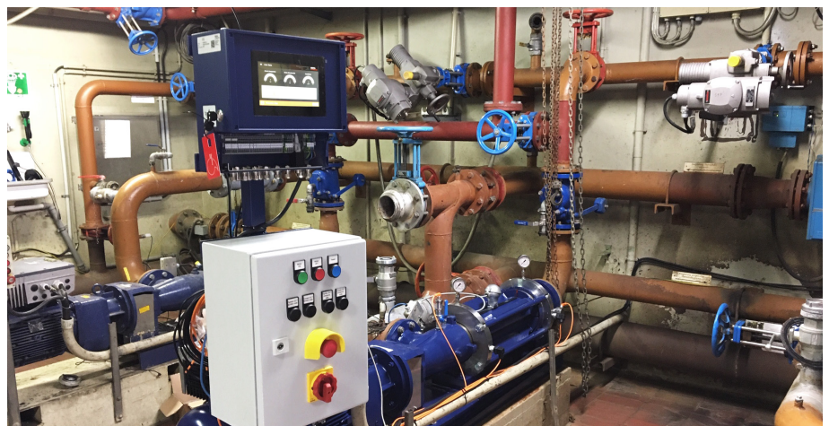
Installation of BN 35-6LAS including SEEPEX Pump Monitor at the plant.
